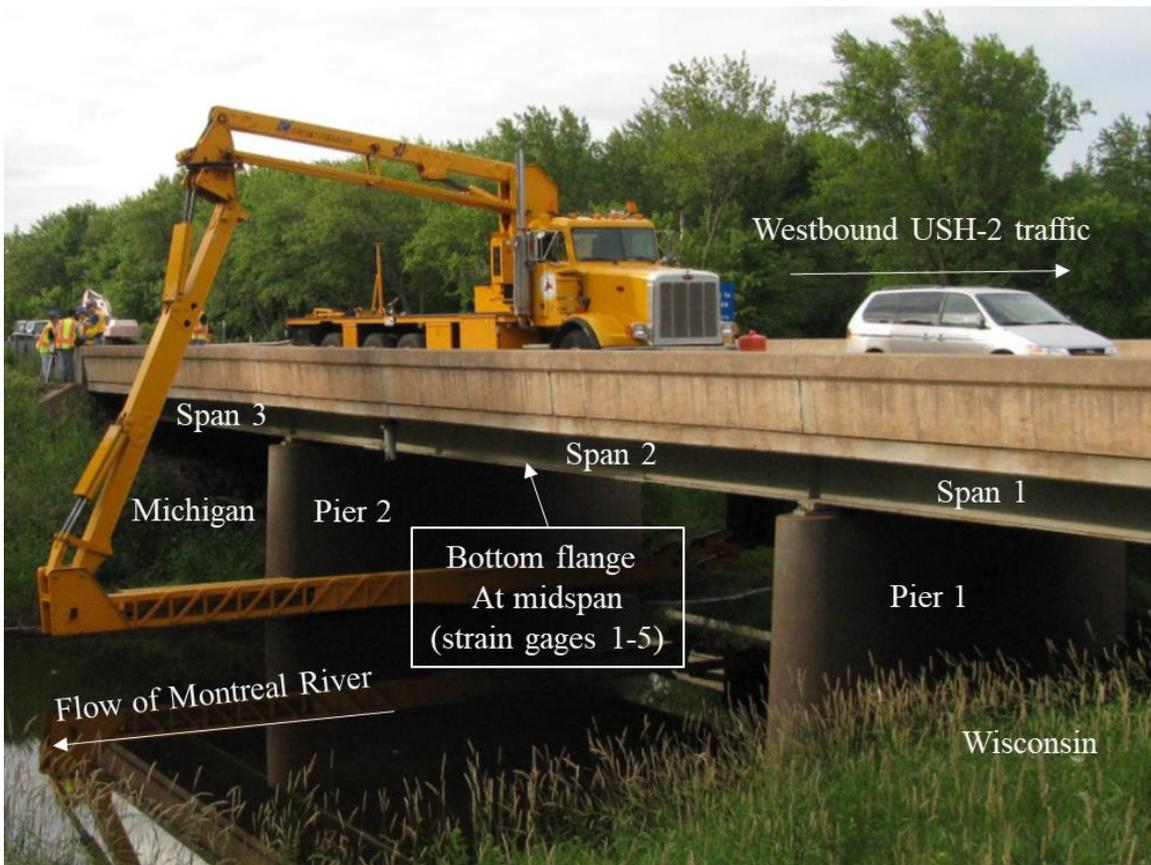
Figure 1.16: bridge configuration and location of SHM sensors on the bridge.
