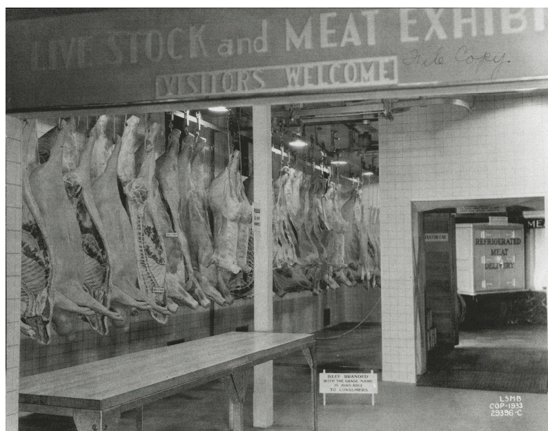
Figure 3.3. Packinghouse cooler. Source: Photograph no. 29396-C COP-1933; RG 16-Ex-52; NACP.
