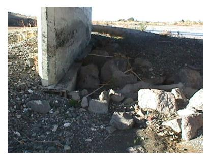
Figure 1: Scour pocket along, rather than at the upstream or downstream end of, a bridge pier
