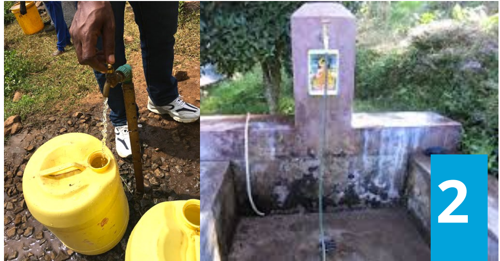
Public tap/standpipe: Public water point, has one or more taps constructed from brick, masonry, or concrete
