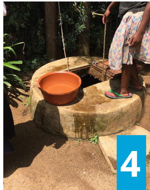
Protected dug well: Dug well protected by runoff by a well lining or casing raised above ground level and a platform that diverts spilled water away from the well
