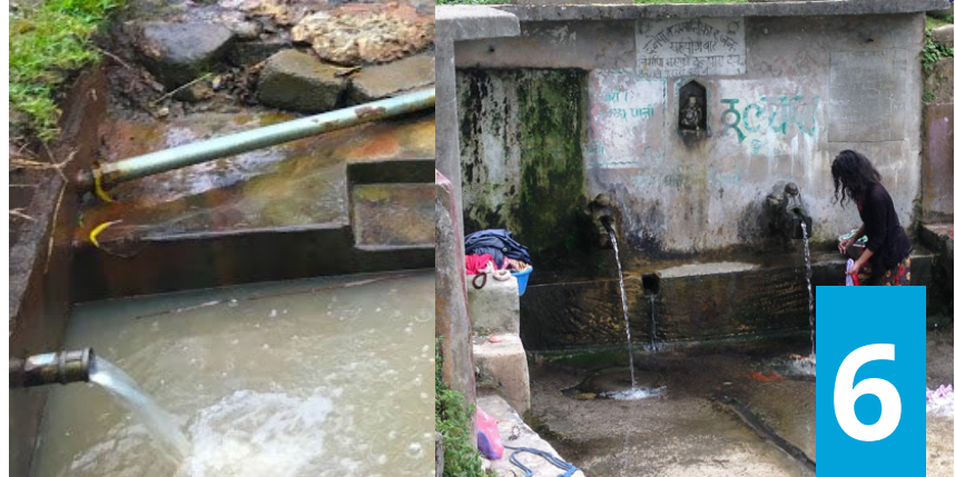
Protected spring: Natural spring is protected from runoff and contamination by a "spring box" constructed of brick, masonry, or concrete built around a spring so that water flows directly out of the box into a pipe or cistern
